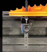
17. Check that the brackets are aligned at 90° to the platform planks, then tighten the nyloc nuts on the channel bolts sufficiently to ensure that both bracket assemblies are securely fastened to the platform and cannot move.
