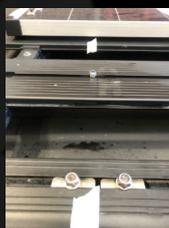
11. Slide the 2 remaining channel bolts (**Part C**) into the channel/slot of the first full plank from the edge rail, locating them roughly opposite the corresponding channel bolts from **Step 10**.
